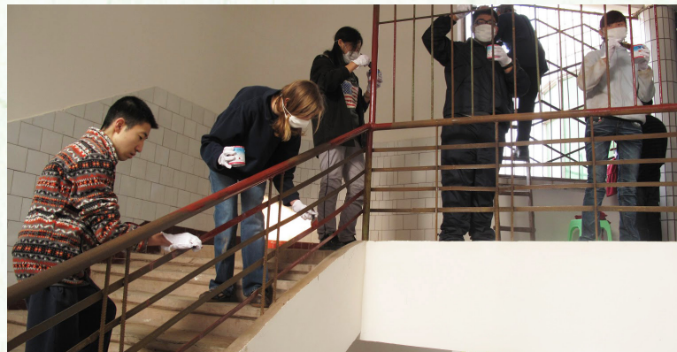
耀中學生參與簡單的翻新工程 YCIS students carry out the refurbishment project
